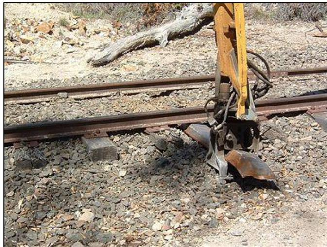
Figure 4. – Steel sleeper being inserted in track
