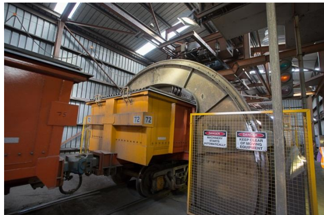
Interior of tippler shed
