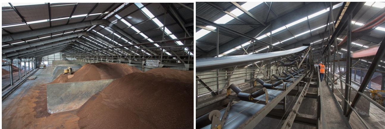
Figure E.2 : Burnie bulk materials shed interior
