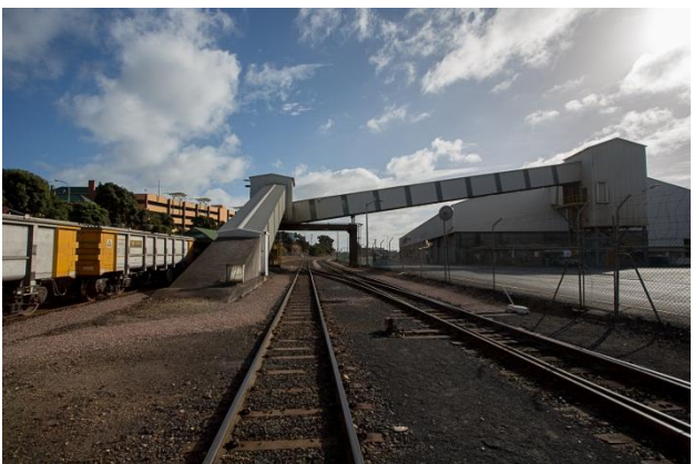
Elevator conveyors from tippler to bulk mineral shed
