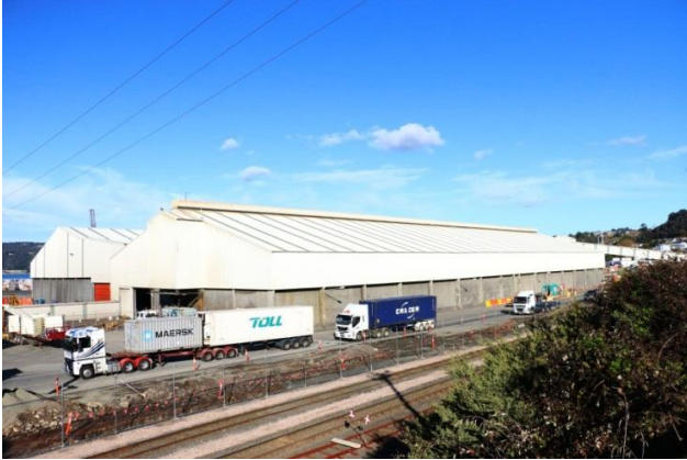
Bulk minerals shed
